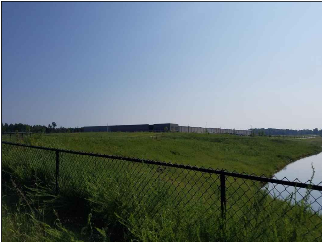
Figure 5.28. Showing location of previously recorded structures that were demolished during construction of Innovation Way, the retention pond, and the manufacturing facility, facing northeast.
