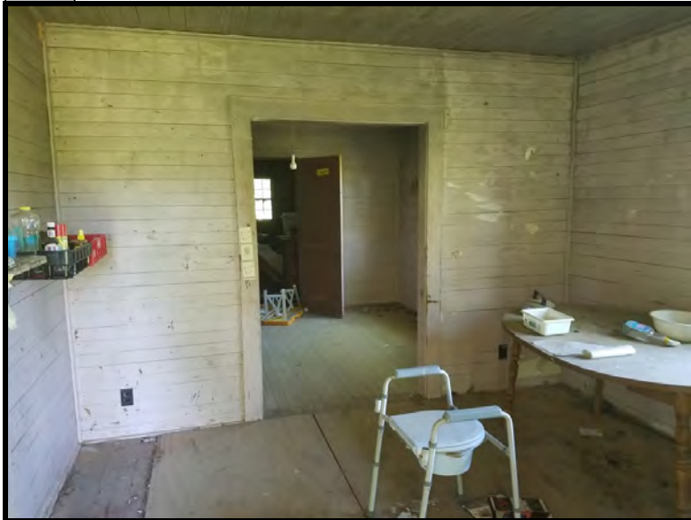
11 Interior view of the on-site residence.
